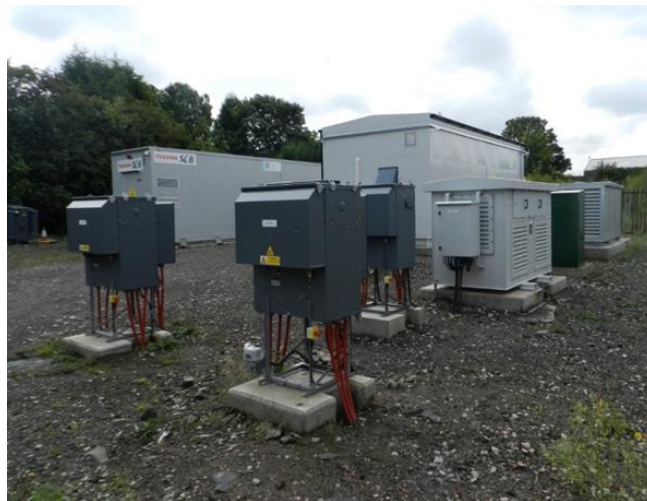
Fig. 3. Site Photo – showing battery system on the left and the inverter on the right with air handling unit
