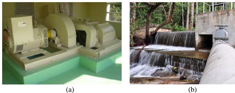
Fig. 1. (a) Hydropower generator of the Tapnakorn hydropower plant project, Chanthaburi province in Thailand to power set up 35 kW, speed 1,500 rpm, efficiency 94 %, (b) weir due to water conservation in community village area.
