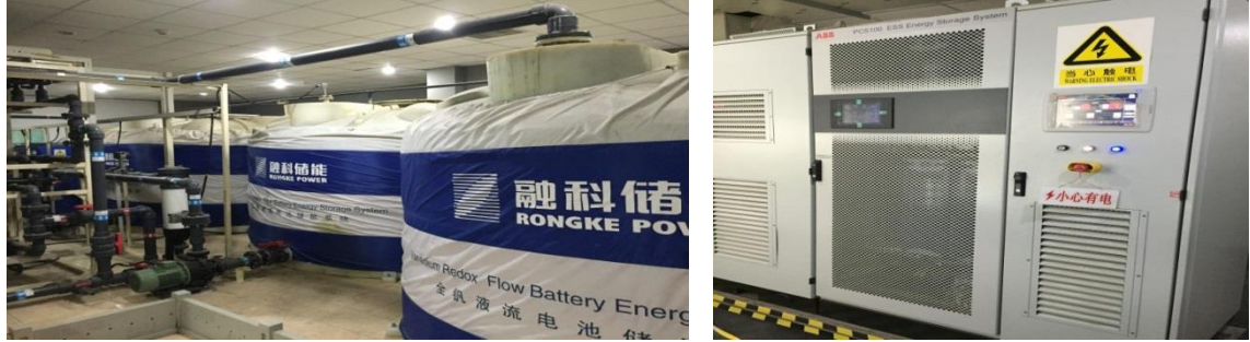
Fig. 4. VRB (left) and the PCS (right) installed in the test facility.
