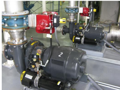
Fig. 9. Rentricity flow-to-wire installation, Keene, NH.
