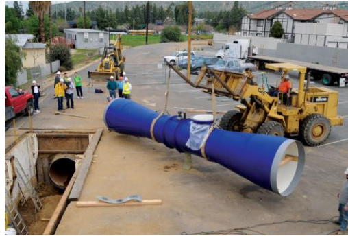
Fig. 8. Lucidpipe installation in Riverside, California.
