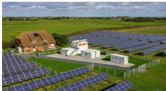
Fig. 5. Central “Tribrid Power Plant” with CLIB, CRFB, PVS, WT and local control center.
