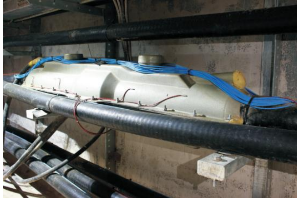
Fig. 6. Temperature detection subsystem using optical fibres
